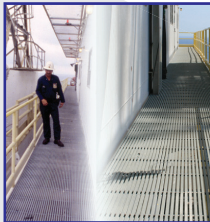
A FRP walkway on an oil rig after 35 years of being in-situ. Fire resistant and durable, made with phenolic resin. Courtesy of Pipex px
