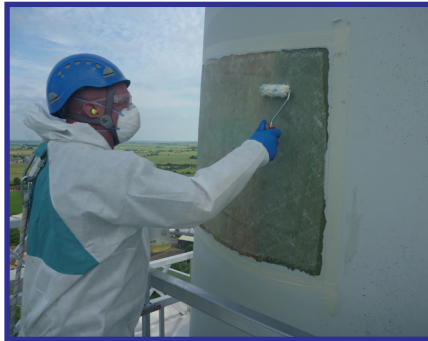
Repair of a wind turbine. Courtesy of Renewable Advice
