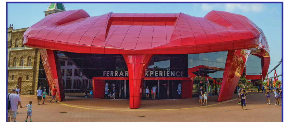
Buildings and rides in the new Ferrari Land theme park near Barcelona use FRP composites cladding and roofing. The FRP parts were moulded using Scott Bader's ATH filled Crestapol® 1212 resin to meet stringent Euroclass fire performance ratings with excellent mechanical performance. Courtesy of Scott Bader
