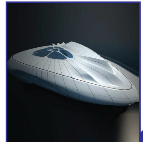
Chanel Pavilion designed by Zaha Hadid comprising of 400 complex curved FRP façade panels. Courtesy of Arup
